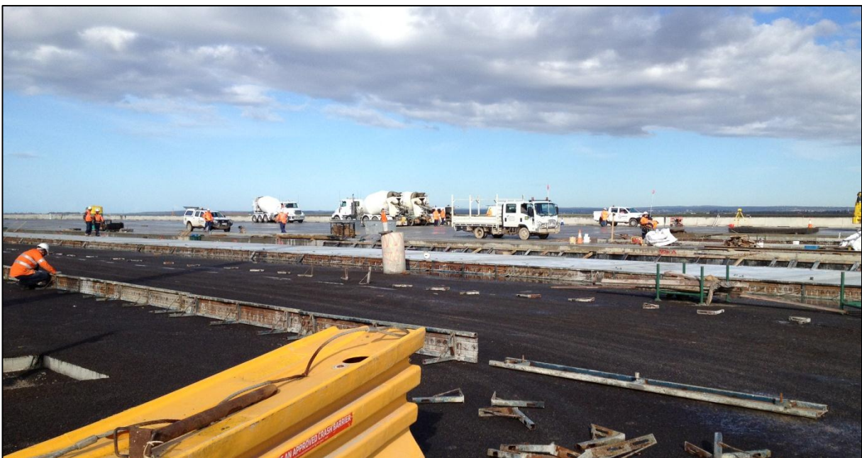
Concrete works being undertaken on the quay side of the new terminal.
