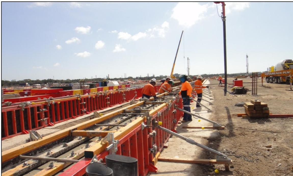
Formation of the ASC rail beam
